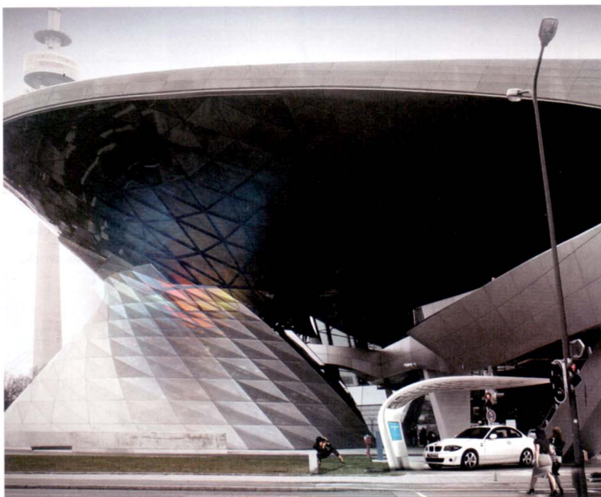
Design proposal for the planned charging station at BMW Welt in Munich (© BMW Group und EIGHT)
